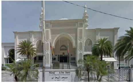
Figure 1.1 Masjid Al Bukhary, Kuala Lumpur.
