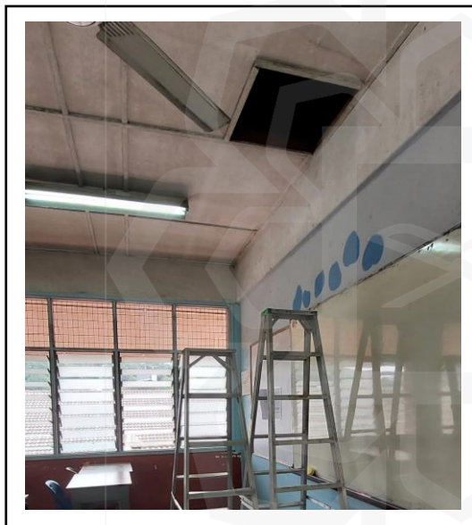
Figure 5.6 (b) SMKSP-B2: Openable Ceiling
