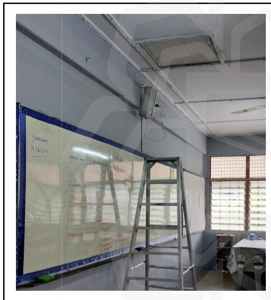
Figure 5.4 (b) SMKTM-B2: Openable Ceiling
