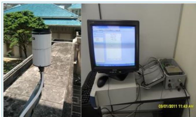
Figure 3.10. Rain gauge installation site and data logger
