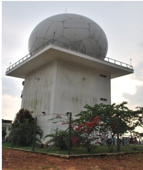
Figure 3.9: MMD Radar Station at Bukit Tampo, Selangor, Malaysia
