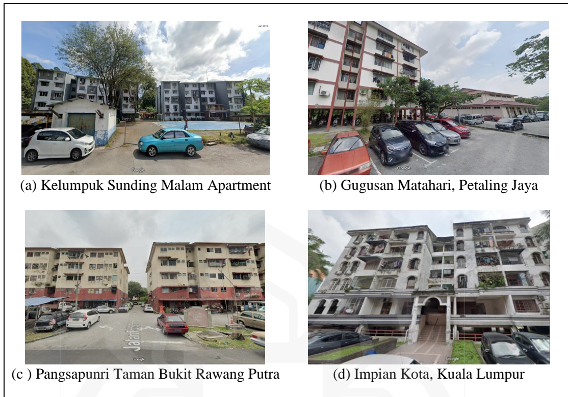
Figure 3.3 Examples of low-cost strata housing (walk-ups)
