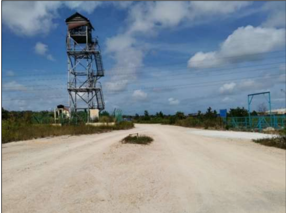
Figure 3.3 Observation tower and tube well.
