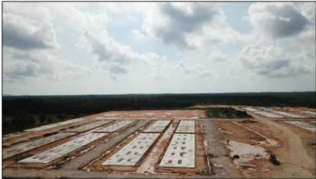
Figure 15. Aerial view Priya construction site 1
