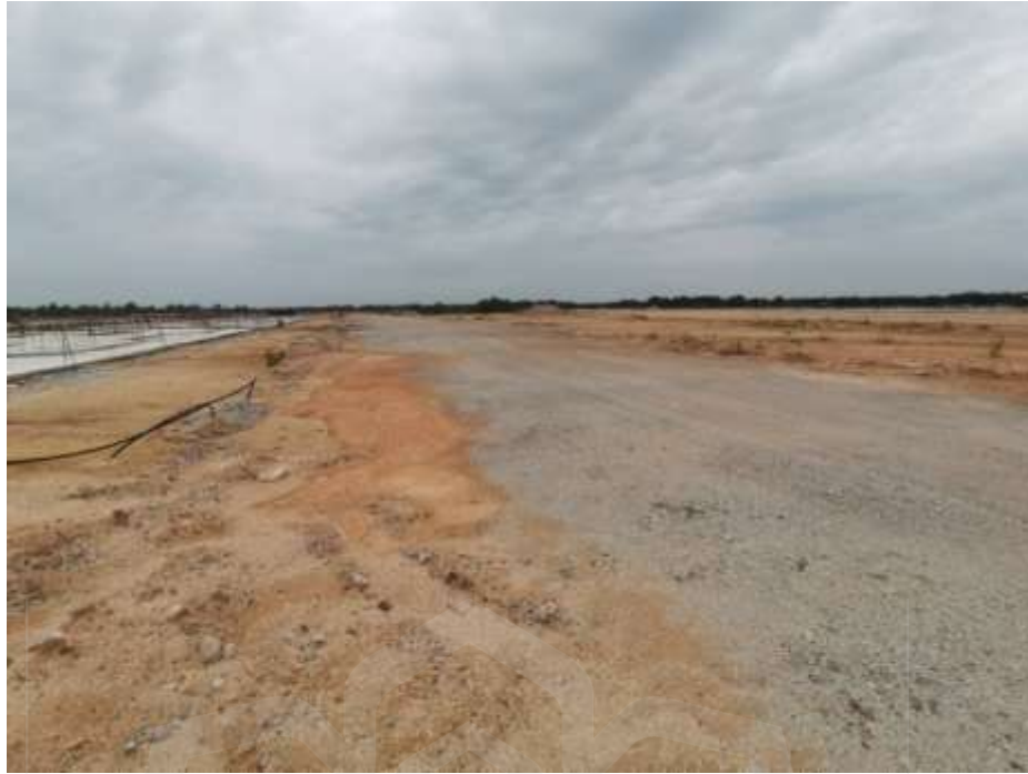
Figure 5.18 Crusher run acts as a temporary road at the construction site.
