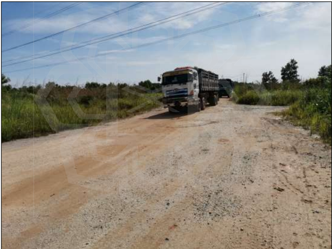
Figure 3.13 The dump tracks enter the construction site.
