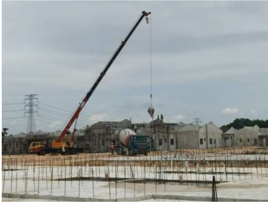
Figure 5.19 Concreting and cementing in progress during dry weather.
