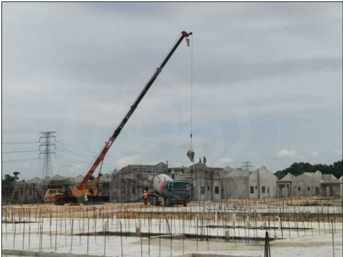
Figure 3.14 The raft foundation and superstructure in progress at the construction site
