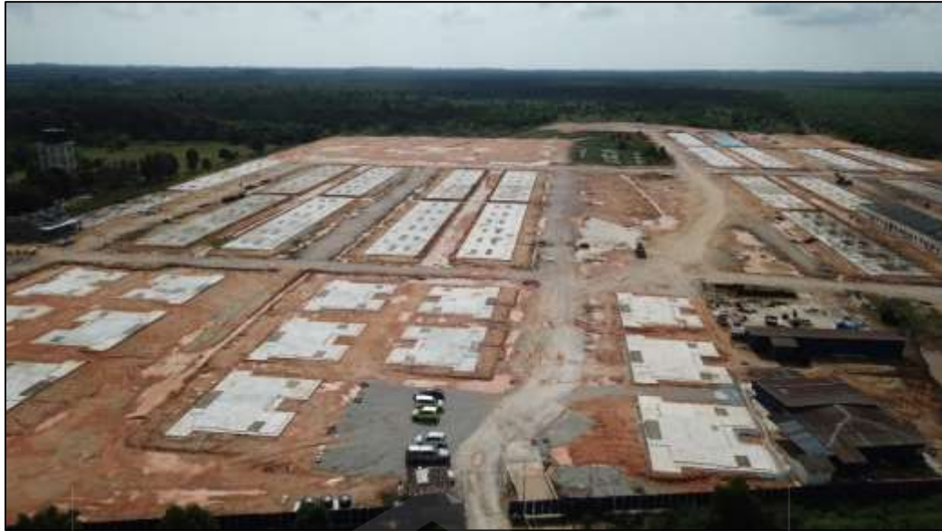
Figure 5.16 Foundation condition at the construction site on 12 th June 2020.
