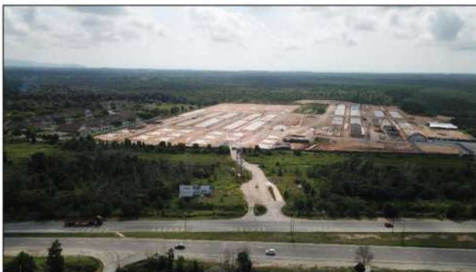
Figure 17. Aerial view Priya construction site 3
