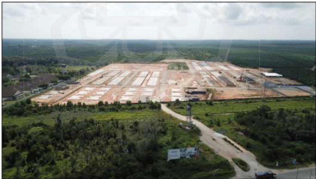
Figure 16. Aerial view Priya construction site 2
