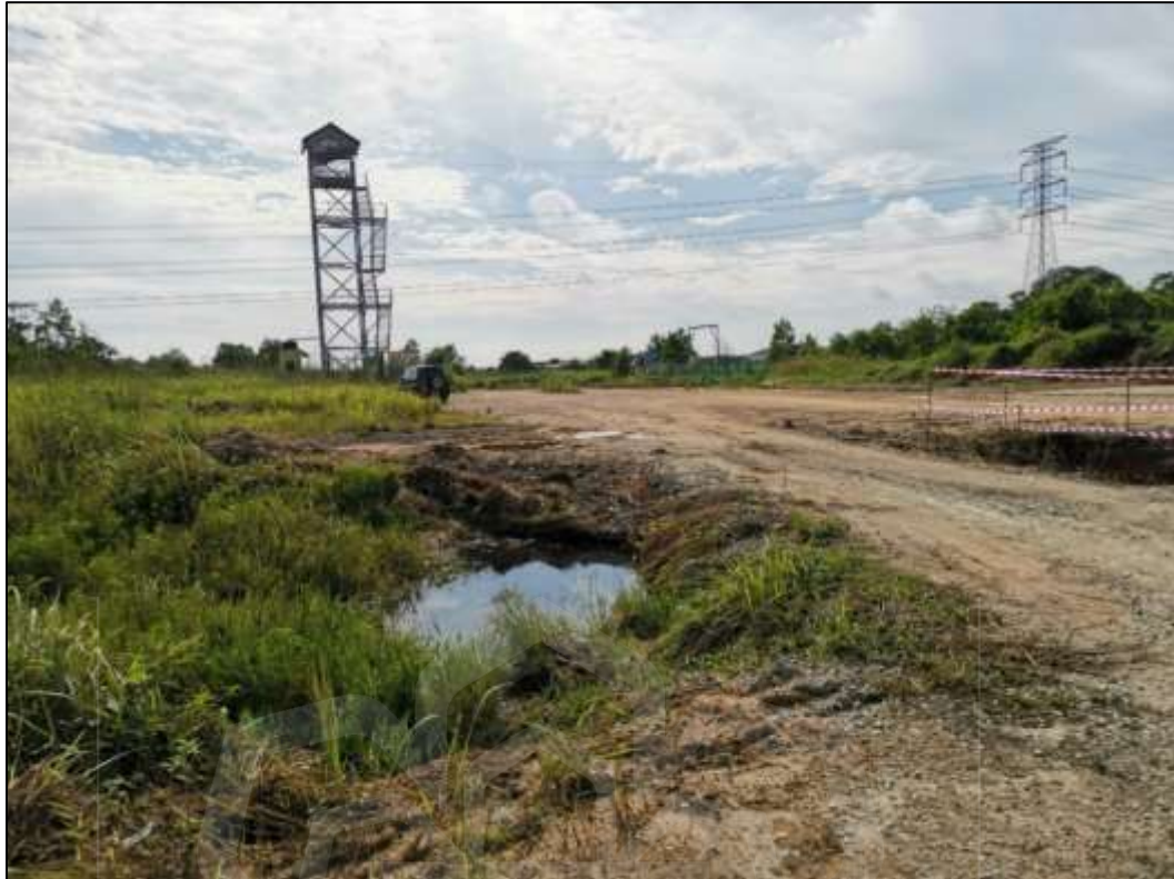
Figure 3.10 Soil and gravel unpaved road. The temporary road is not unpaved as the project site is still under construction.
