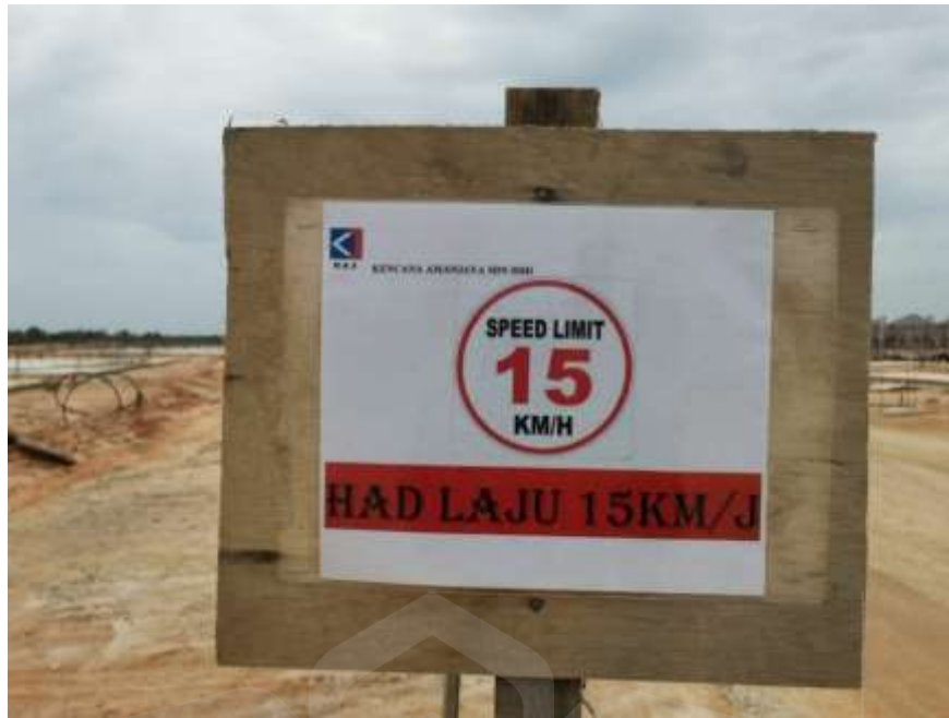
Figure 5.17 Signage speed limits at the construction site.
