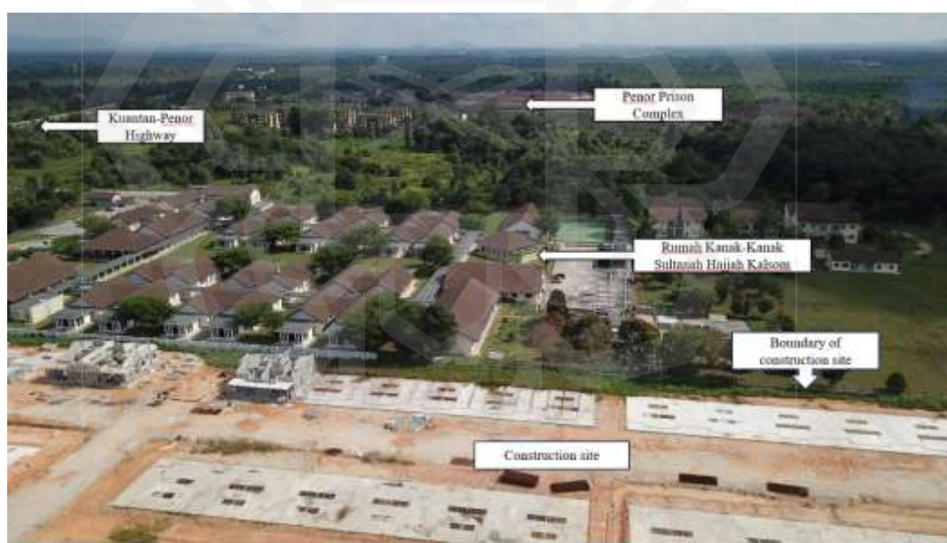
Figure 5.20 Borderline between RKKSHK and the construction site.
