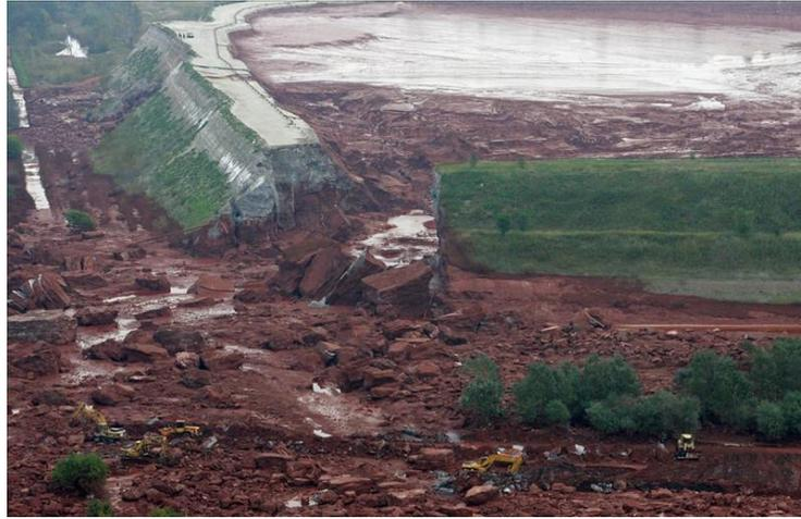
Figure 2.3: The Crack Dam Corner causing the Alumina Spillage at Ajka, Hungary in 2010 (Turi et al., 2013)
